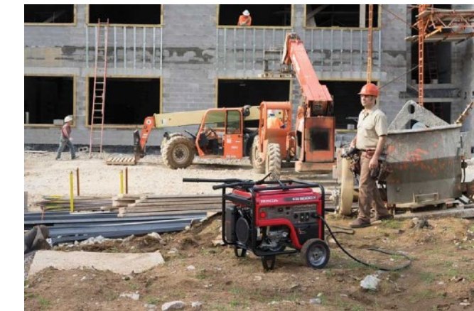
Generators & Emergency Power
